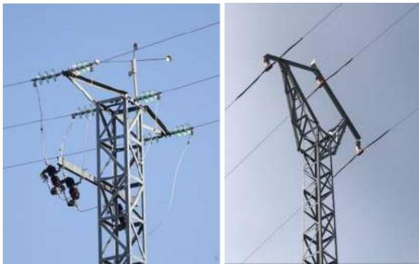
Figure 9 – Several types of perching and nest deterrents.
