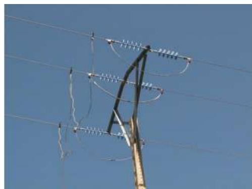
Figure 7 – Increase of insulator chains.
