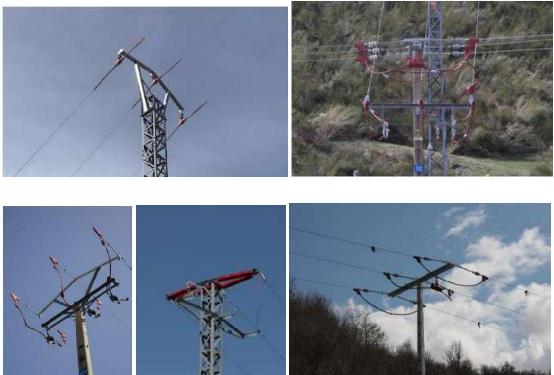
Figure 6 - Insulators against bird electrocution.
