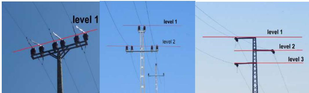
Figure 1 – Examples of three types of line typology, with different levels bird collision
