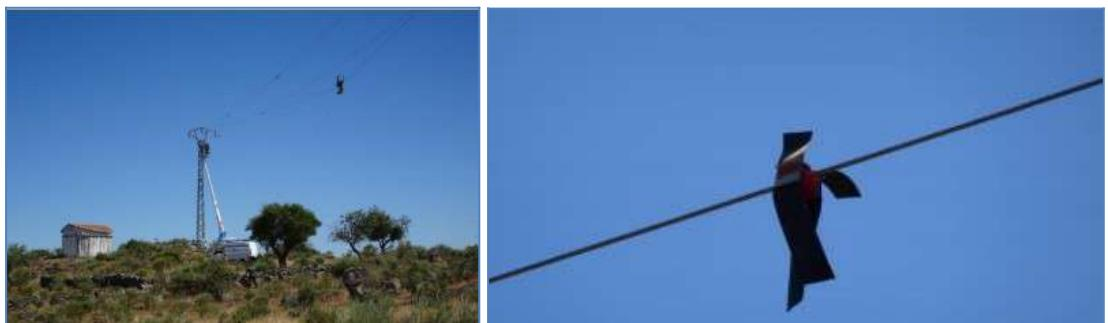
Figure 4 - Bird saving Strips in Xs. placement on the line and device.
