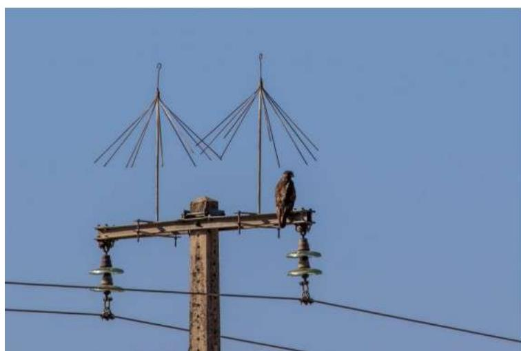
Figure 11 - Common buzzard perched on a cross with umbrella-like deterrent elements on the 20 kV power line. ZEPA Valle del Tiétar Lanzahita, Ávila. July 2019. Photo: Photo: R. Sánchez / Grupo Eco
